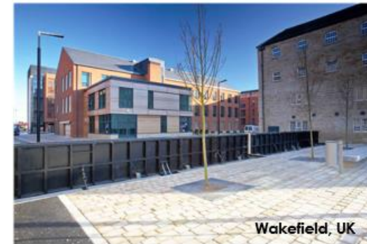
Flip-up flood barriers that can be remotely deployed and incorporated into the street (Image credit: Flood Control International)
