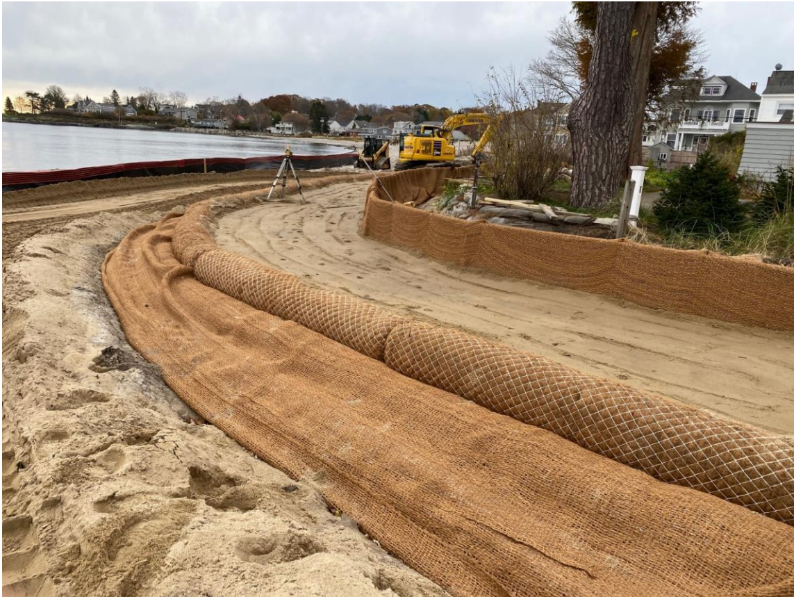
Dune Restoration - Installed by Wilkinson Ecological Design
