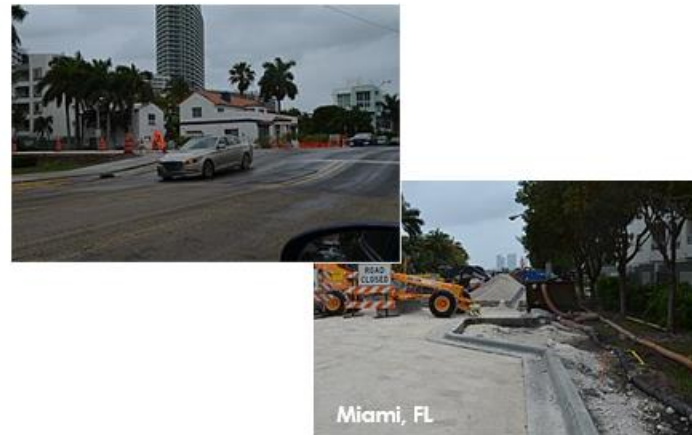
Road raising project (Image credit: CC 1.0)
