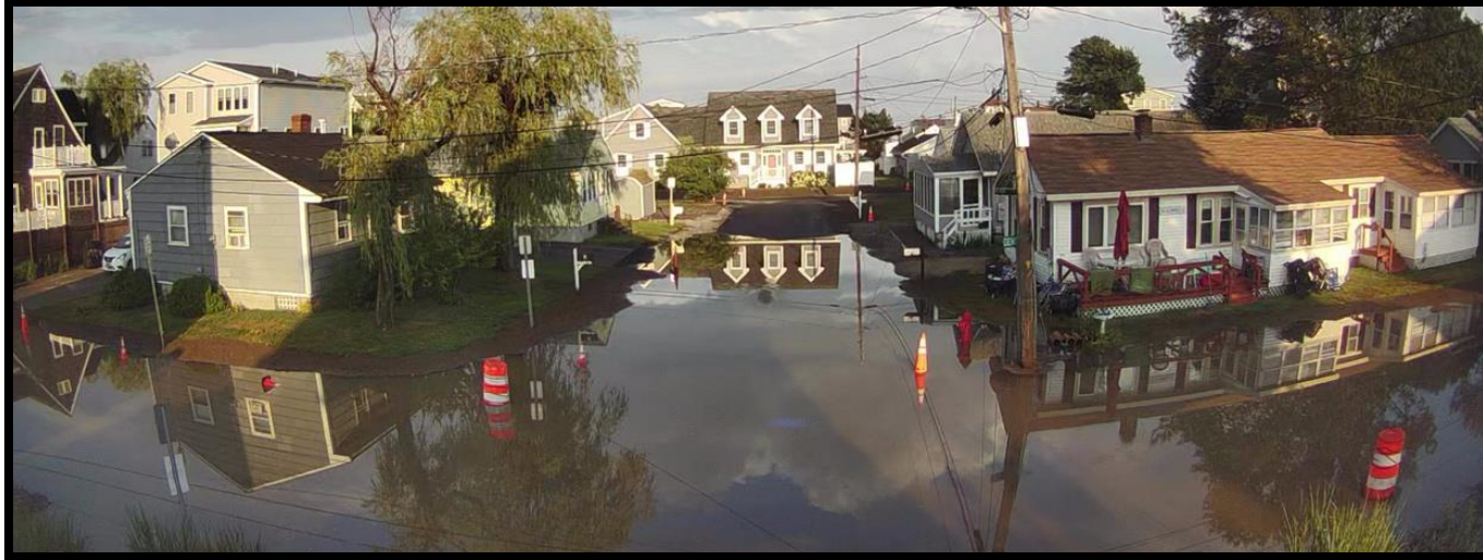
Before pumps were activated
