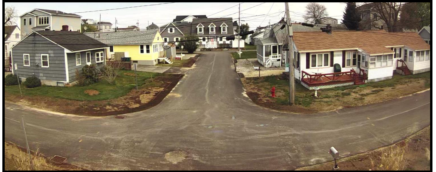
After pumps were activated
