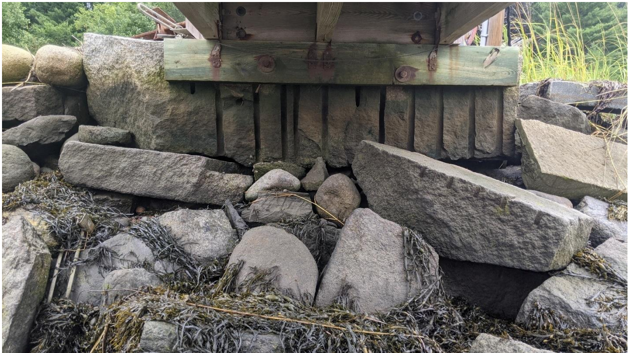
Stone armoring under pier
