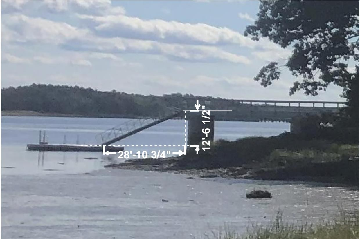
Scaled measurements in the photograph may not be "actual" distances. The photo perspective is skewed relative to the alignment of the pier and dock. However, the scaled measurements are relative to one another and provide an approximate gangway slope.
