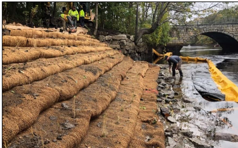
FES with Toe Rock Upper Bank Failure Treatment
