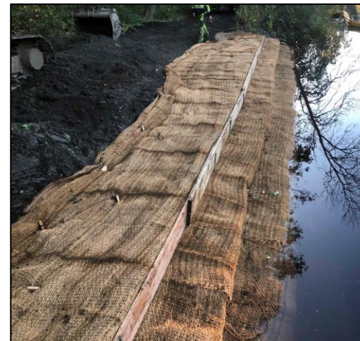
FES with Toe Rock Upper Bank Failure Treatment
