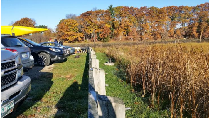
Parking, Guard Rail & Marsh Interface
