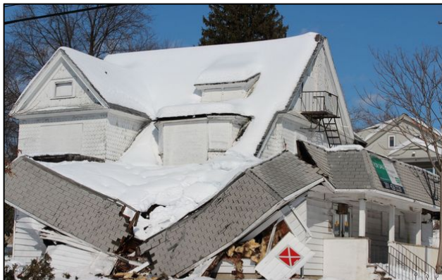
Exceeded design values of snow loads on building roof
