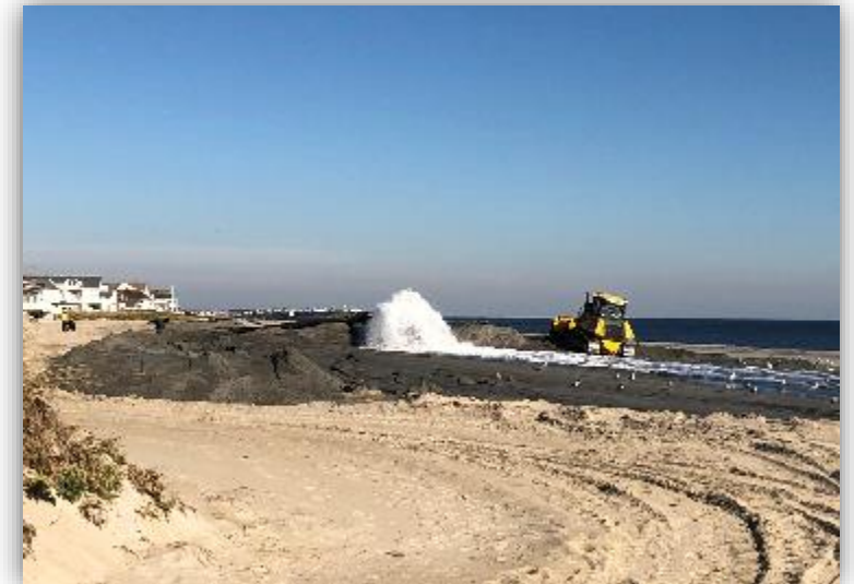
Pipe outlet and Beach Grading
