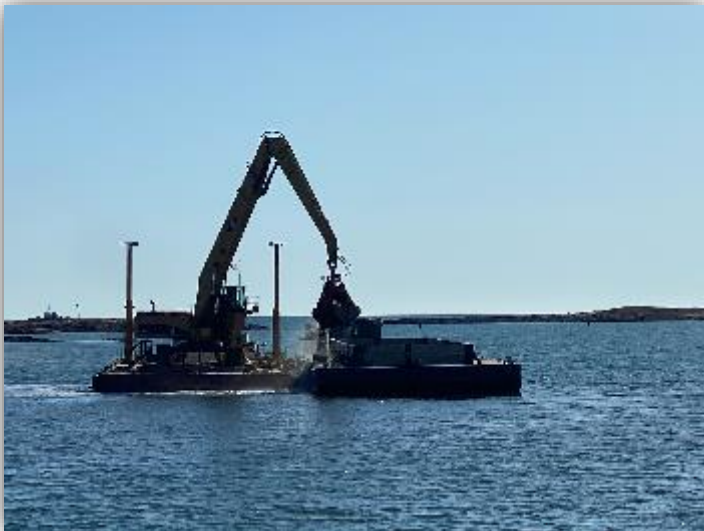
Example Dredge Operation (loading the scow)
