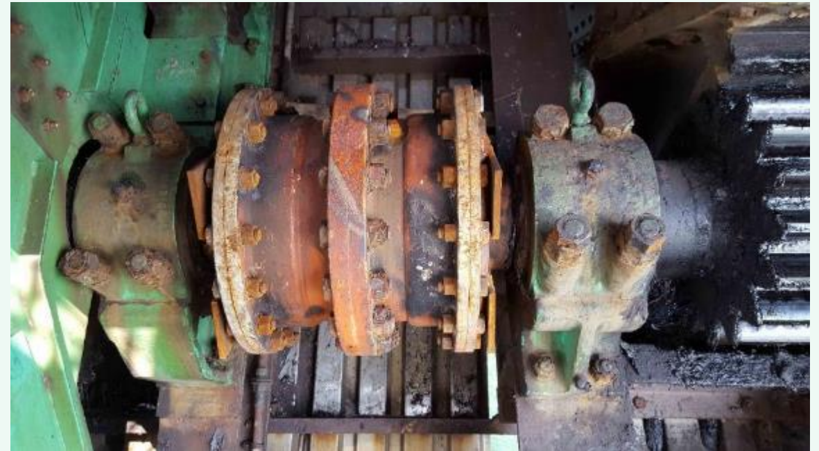
Bascule span coupler
