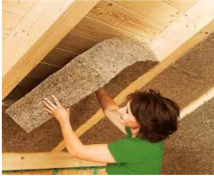
Insulation is wood fiber
