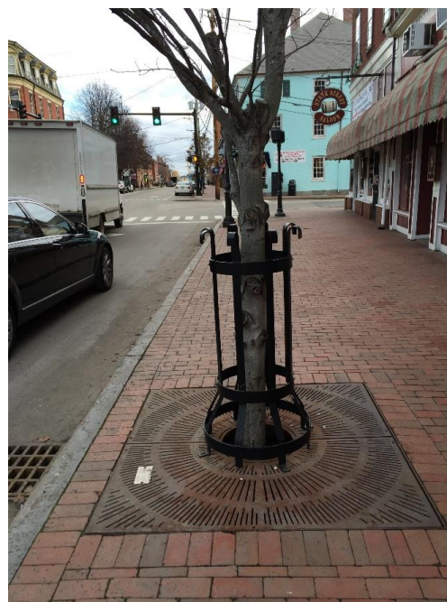
Figure 7: Tree Planter Combined with Catch Basin
