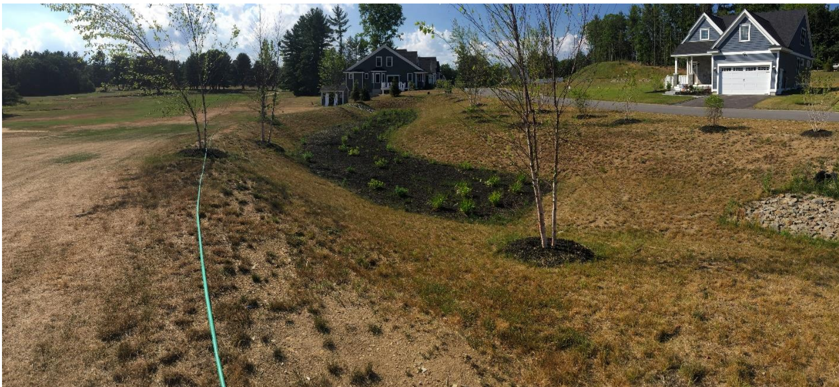
Figure 5-2. A newly constructed bioswale in Rockingham Green for stormwater management and volume reduction
