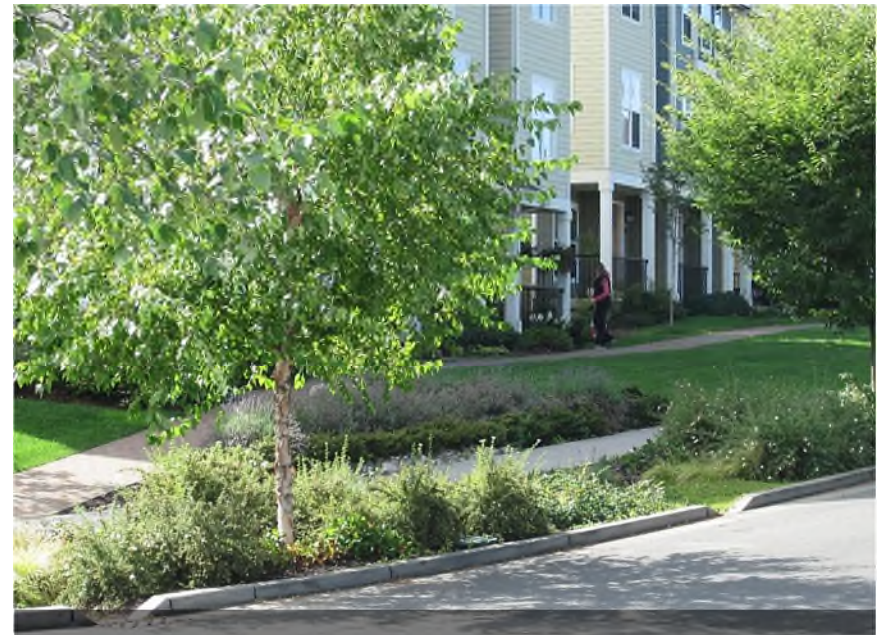
Roadside bioretention can include trees and attractive, low maintenance vegetation to enhance streetscapes.
