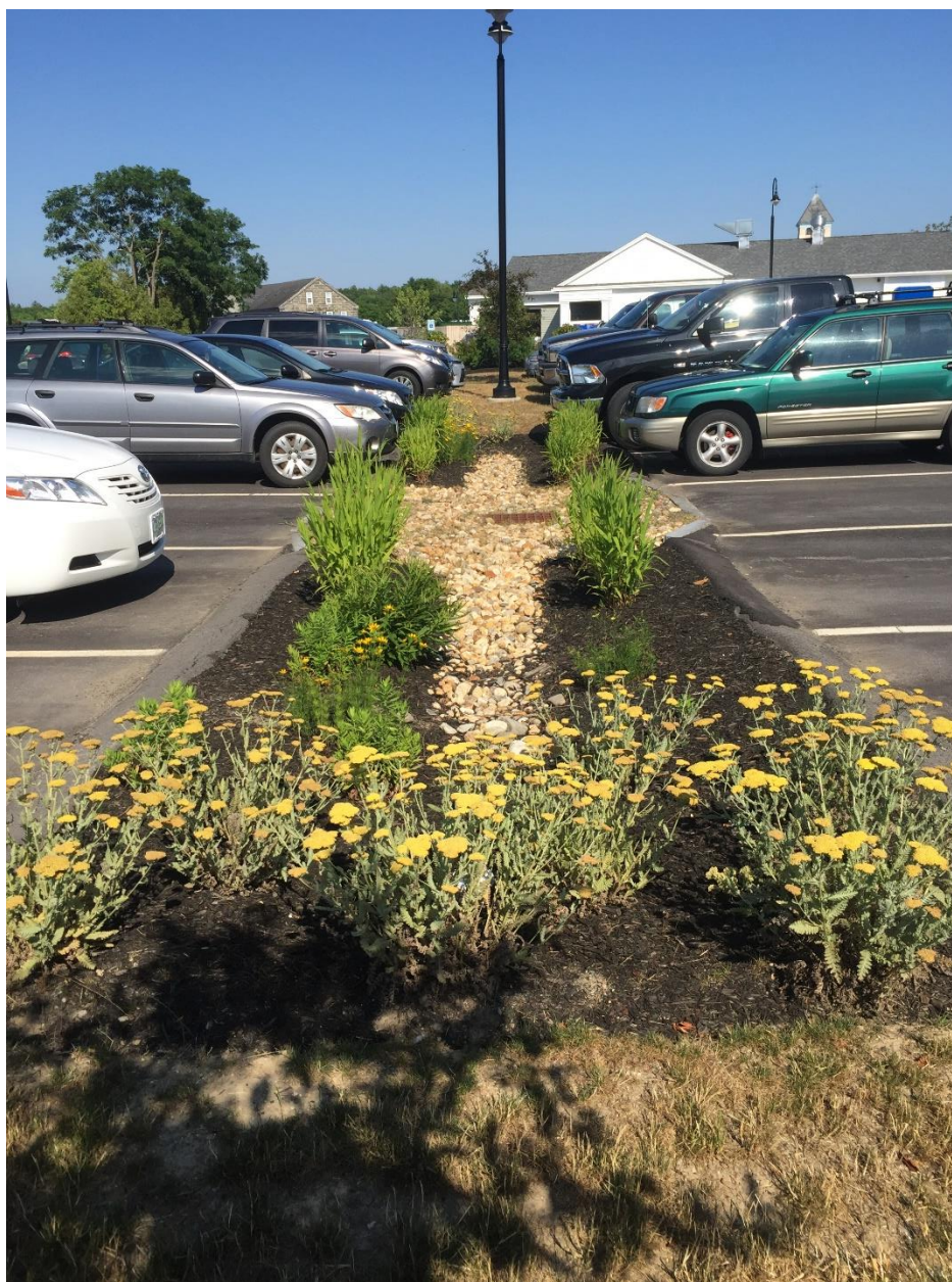
Figure 5-1. Bioswale in Elm Street Plaza
