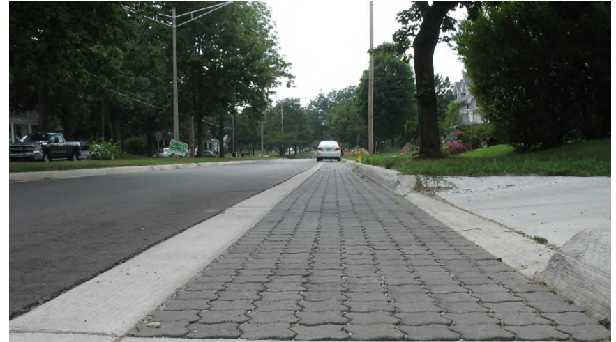
Permeable pavement can be used for lower volume traffic areas such as parking and bicycle lanes. Photo credit: Dan Christian, Tetra Tech, Inc.
